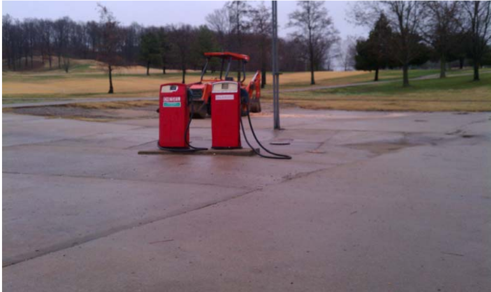
Fuel tanks at Equipment Storage building
