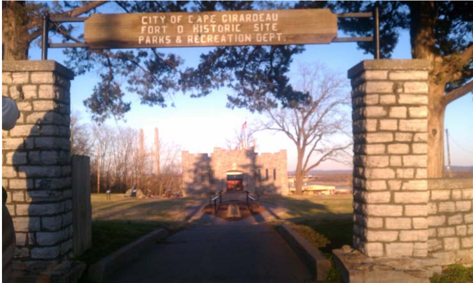
Entry to Fort D Historic Site. The posts used to have lights, which were vandalized and removed. The wires are still in the posts.
